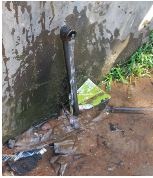
Figure 2: A street tap supplying municipal water to the public free of cost, Netrokona Municipality, September, 2013
