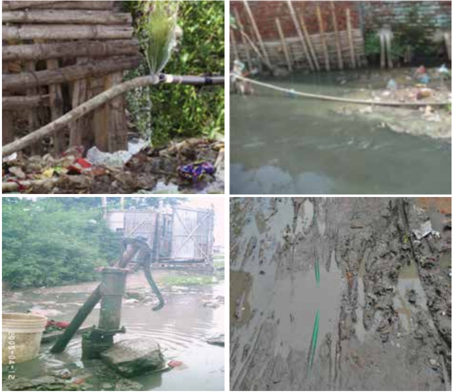
Figure 2: Water distribution pipes near sewage in Dhaka
