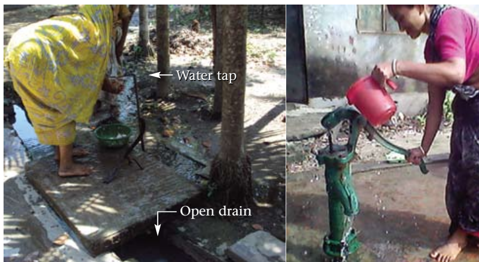
Picture 1: A women washing fish with municipal tap water flowing through a pipeline submerged in an open sewer (left) and a woman pouring tap water into the tube-well to raise water level for drawing tube-well water (right)
