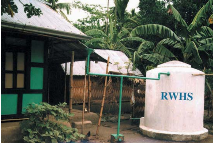
Photo: Household rainwater harvest system used to reduce exposure to arsenic and bacteria-contaminated water sources (Courtesy: Arsenic Team)
