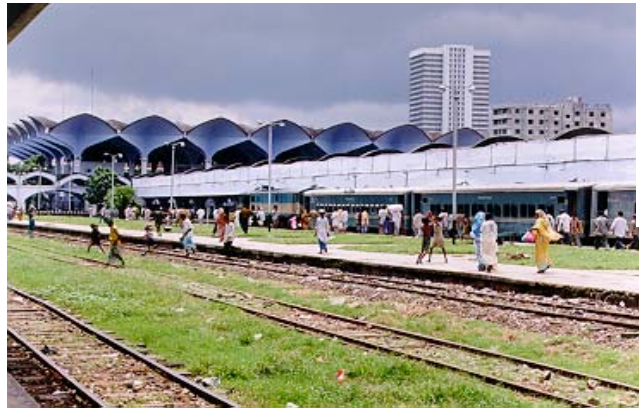
Kamalapur railway station used as significant transit trafficking route
