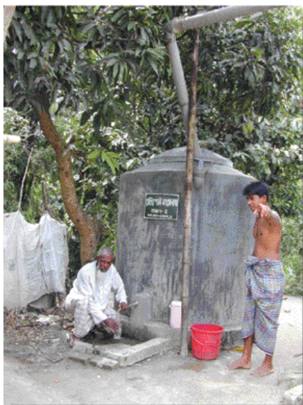
Household-based arsenic mitigation option (rain water harvesting)
